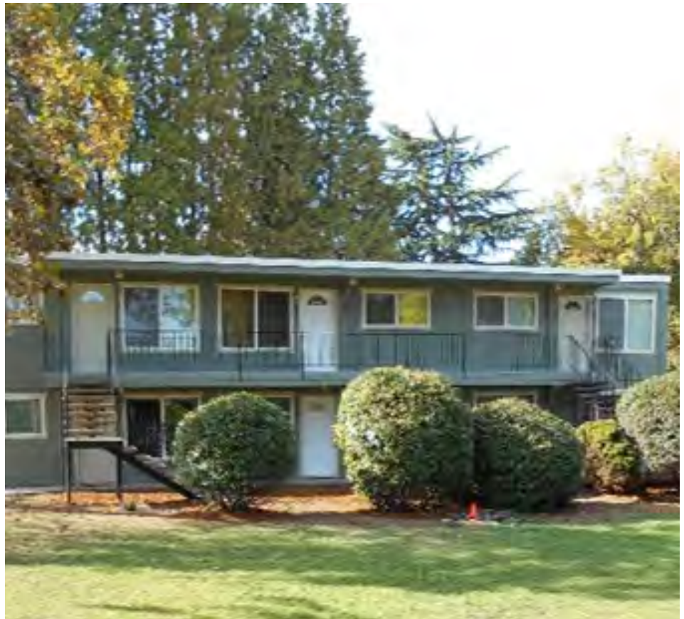
North Polk Street Apartments
