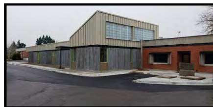
Maintenance Building Expansion
