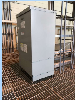
Inadequate lateral bracing or anchoring
