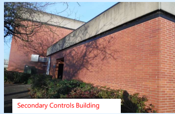
Secondary Controls Building
