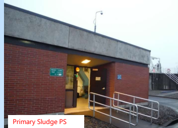
Primary Sludge PS
