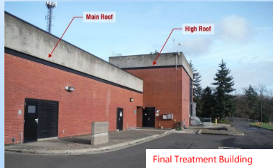
Final Treatment Building
