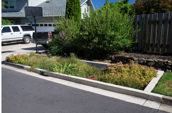
Stormwater Planter can infiltrate and filter stormwater runoff
