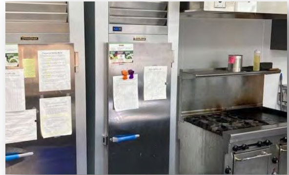
Looking Glass McKay Lodge, Kitchen remodel, Eugene
