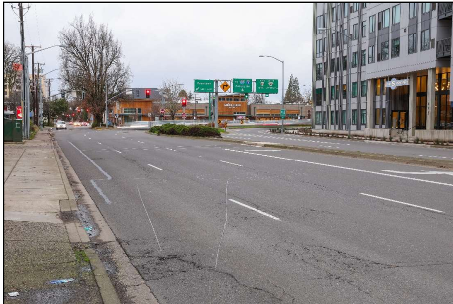
Broadway near Mill Street – Existing Conditions
