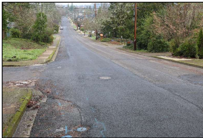
Hilyard Street – Existing Conditions
