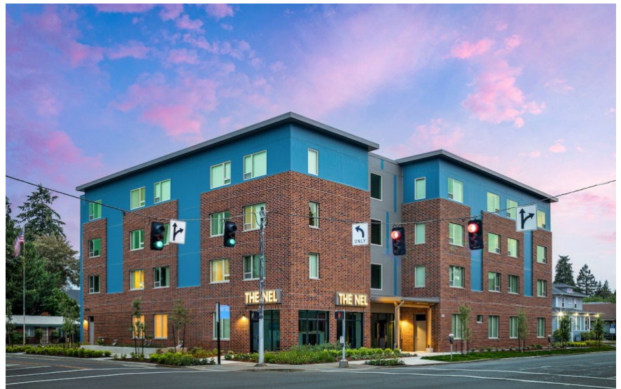
The Nel, permanent supportive housing
