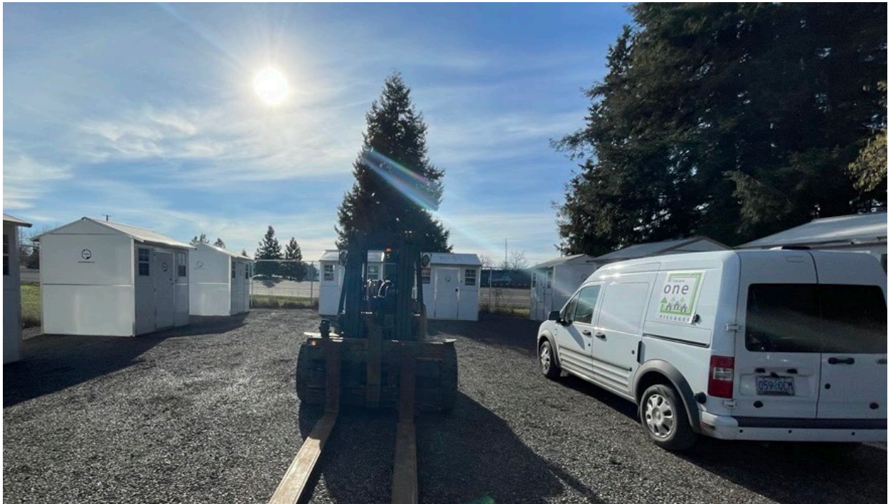
Pallet shelter and infrastructure installation at new City-supported shelter site
