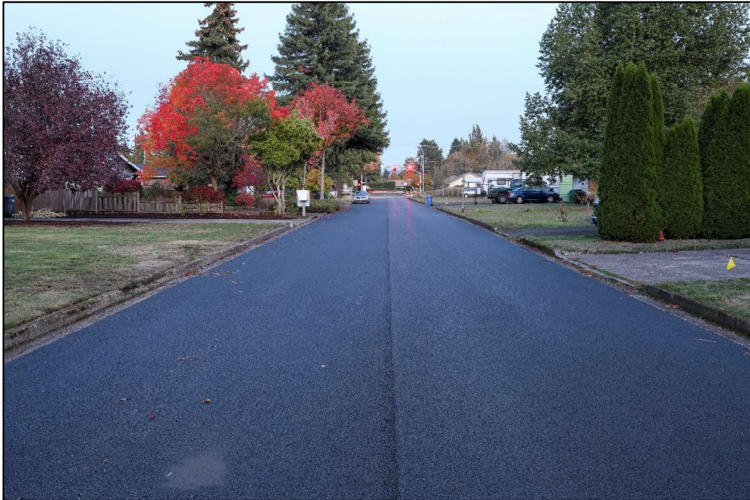
COMPLETED PAVING ON CARMEL AVENUE
