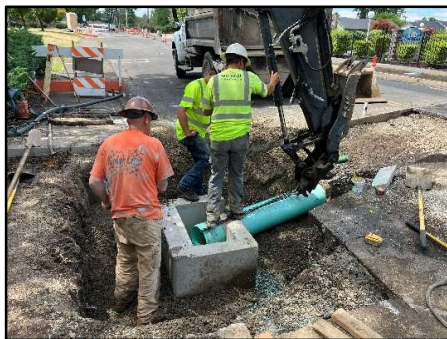
Stormwater Pipe Work on Bailey Lane
