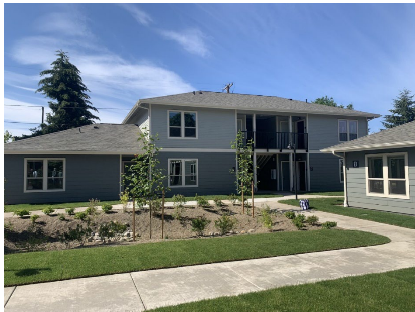
Williams Place, Affordable Housing development for Veterans
