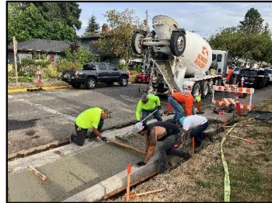
ADA Ramp Under Construction on Carmel Avenue
