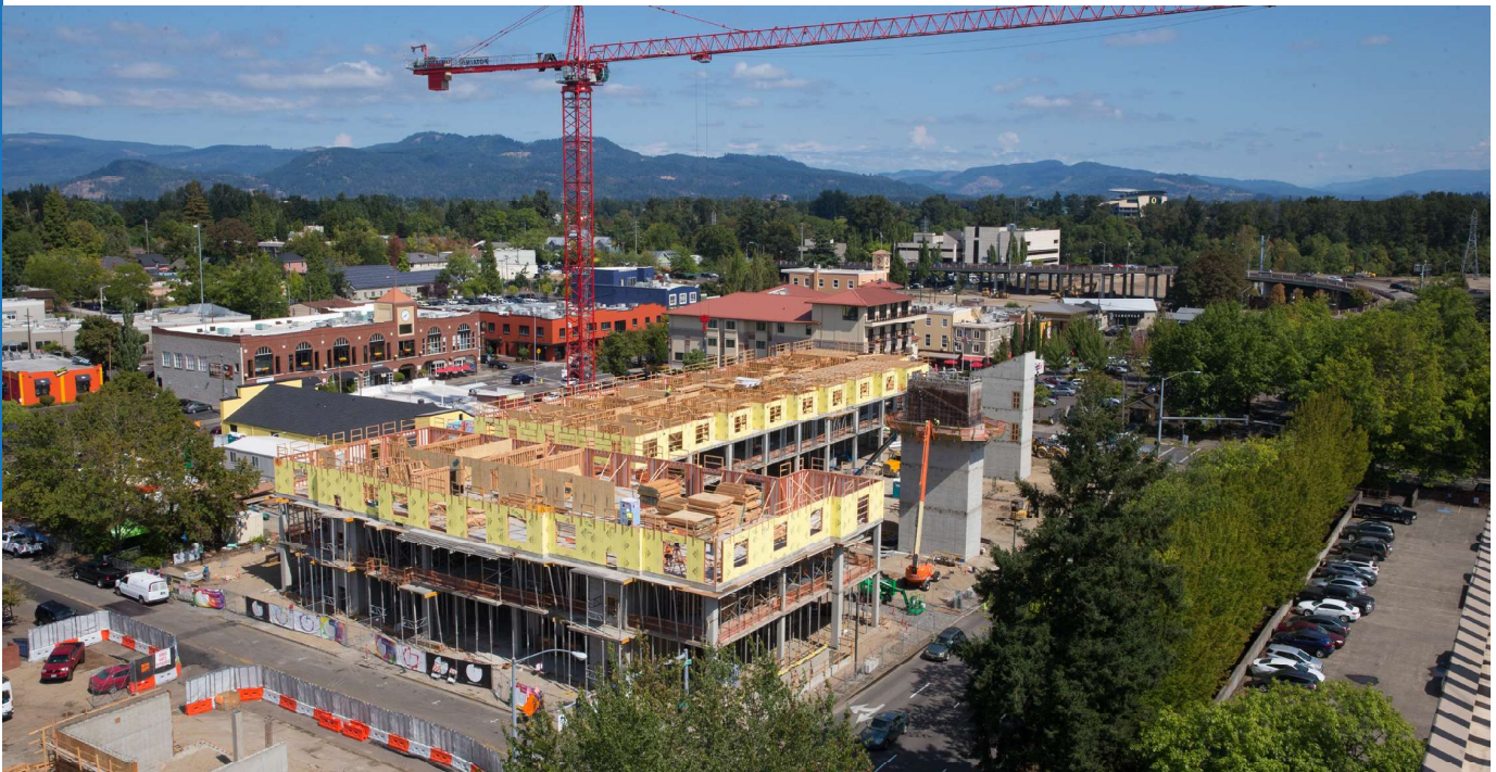
Construction on Gordon Lofts and Hotel
