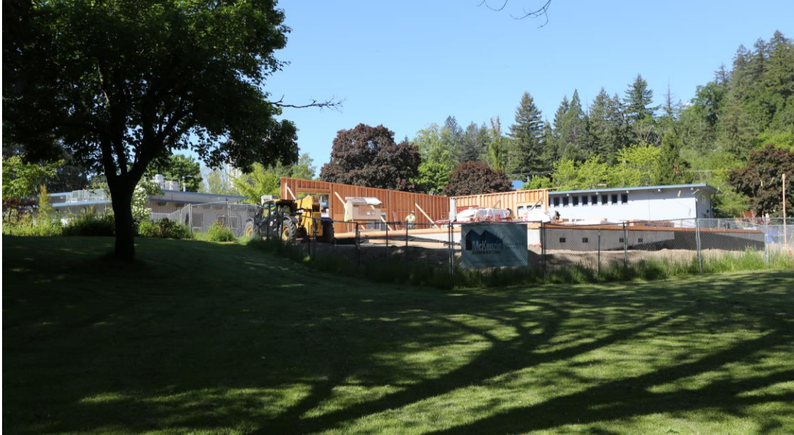
Campbell Community Center
