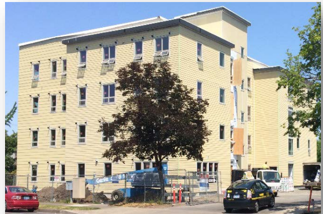
Myrtlewood Apartments, under construction
