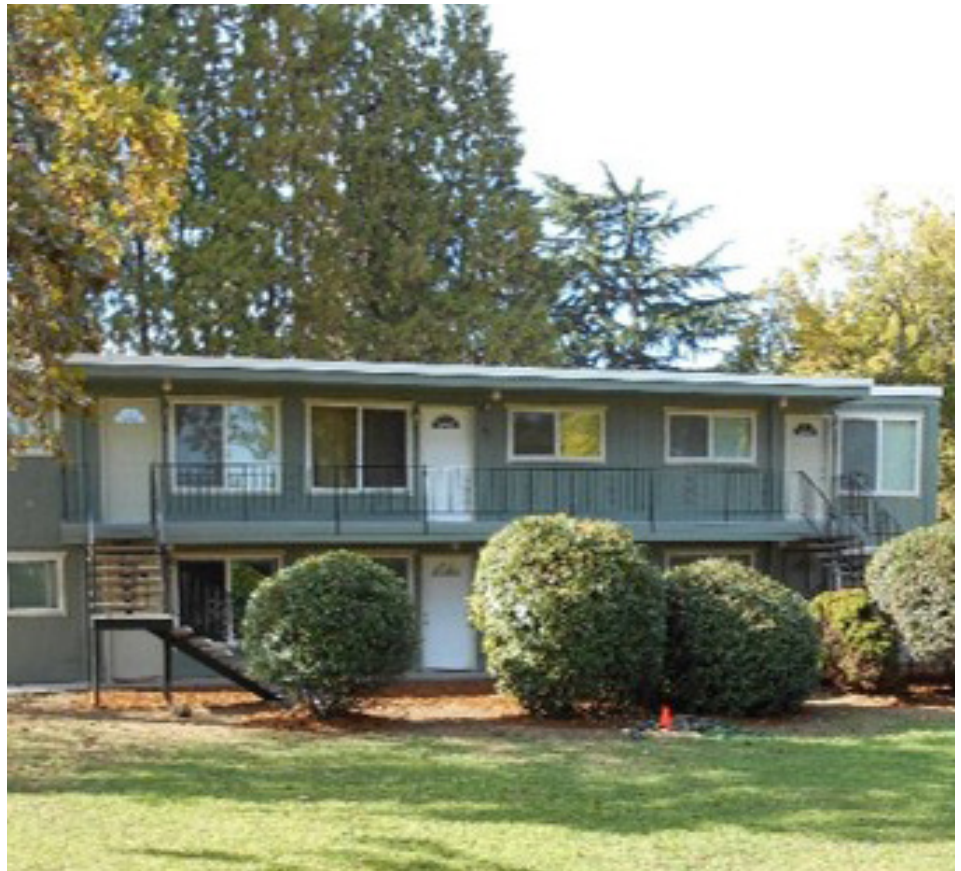
North Polk Street Apartments
