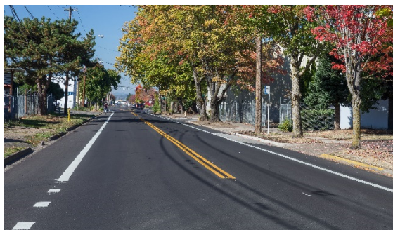
Completed Paving on 2nd Avenue
