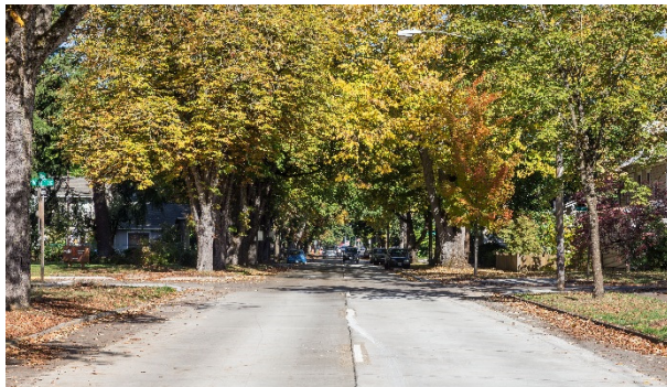
Completed Paving on Jefferson St.
