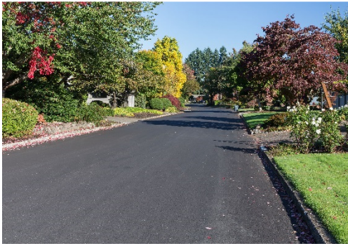
Completed Paving on Tomahawk Ln
