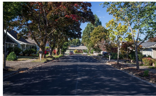
Completed Paving on lone Avenue
