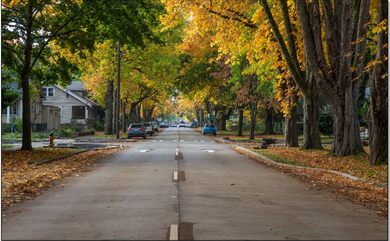
Completed Paving on Jefferson Street
