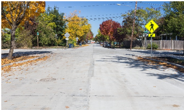
Completed Paving on Jefferson St.
