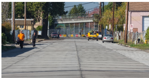
Completed Paving on 1st Avenue
