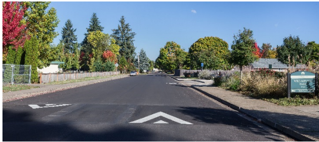
Completed Paving on Best Lane
