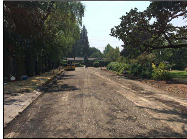
Compacted RAP Base on Pioneer Ct.
