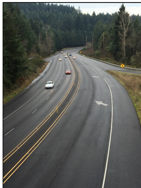
Completed 30th Ave Paving
