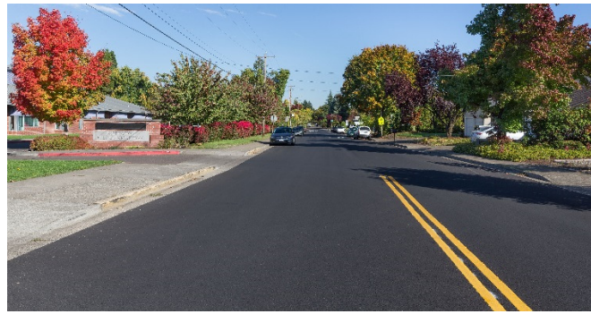
Completed Paving on Calvin St
