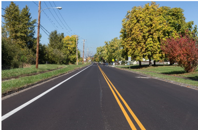
Completed Paving on E. Amazon Drive
