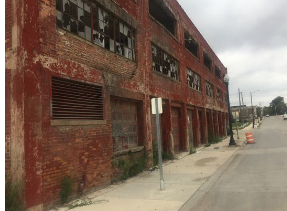
Figure 4: A small glimpse of the Stone Soap Building in its current condition.
