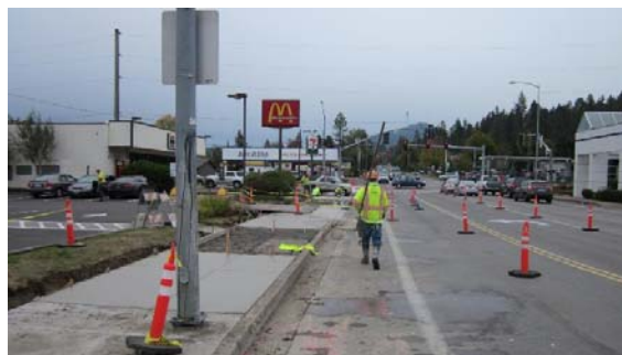
Sidewalk construction north of 29 th Avenue
