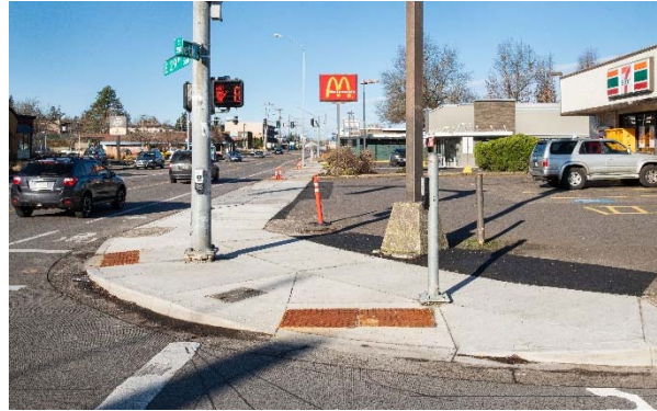
Constructed ADA Ramp on Willamette Street
