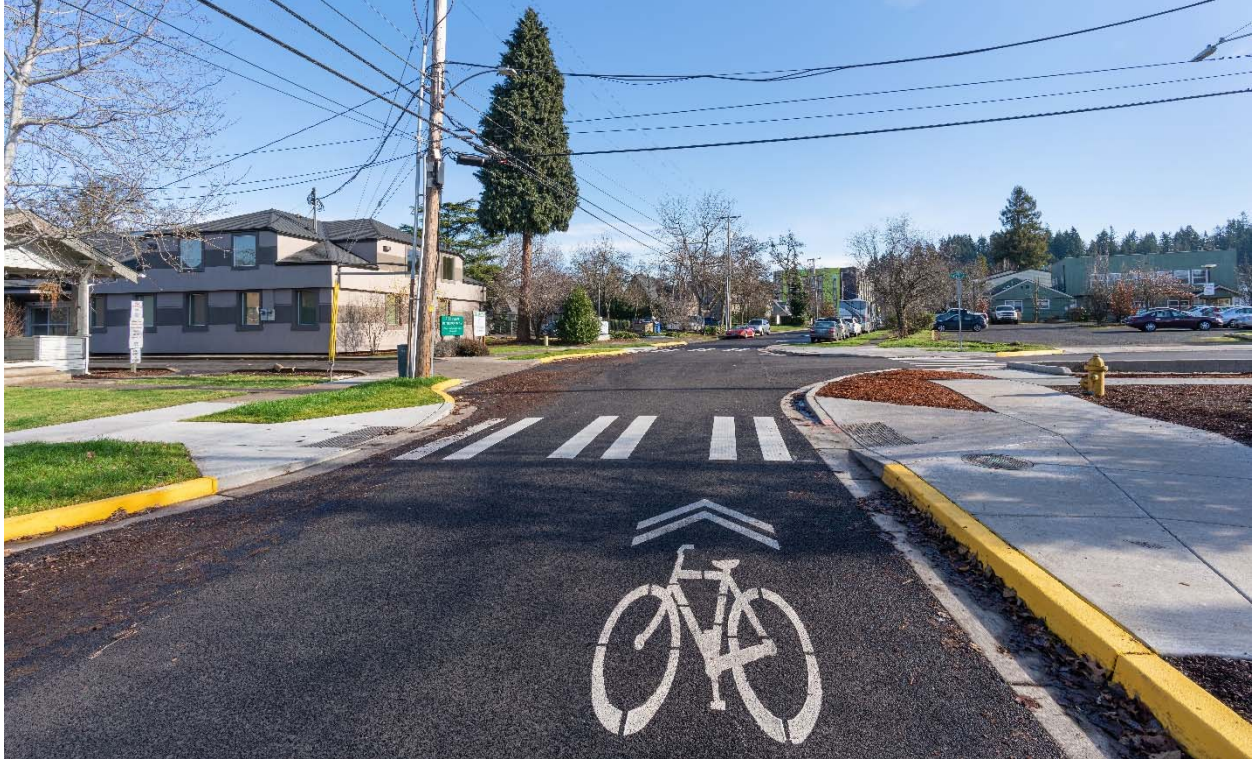
Completed Paving on Garden Avenue
