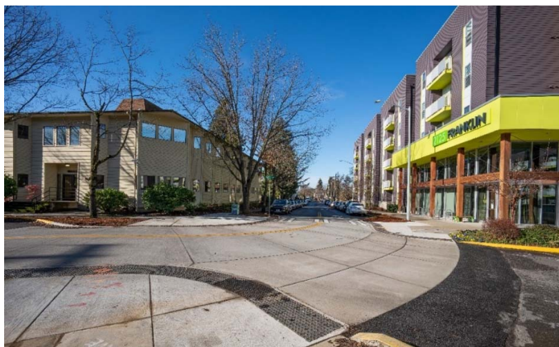
Concrete Raised Intersection at Garden Avenue & Walnut Street
