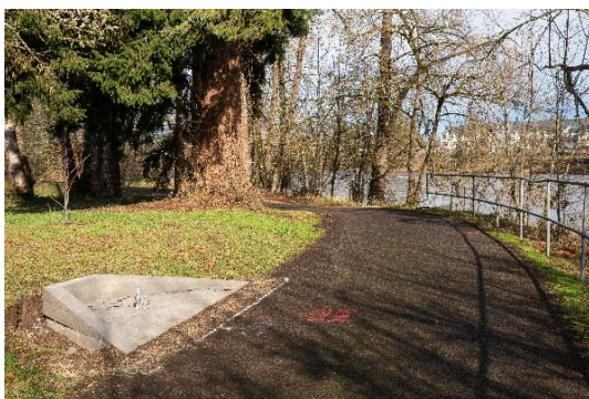
Concrete Light Foundations on the West Bank Path
