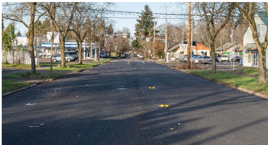
Completed Paving on Polk Street
