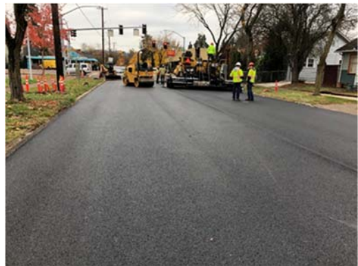
Paving on Polk Street
