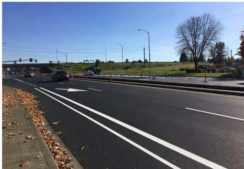
Completed Paving on Barger Drive
