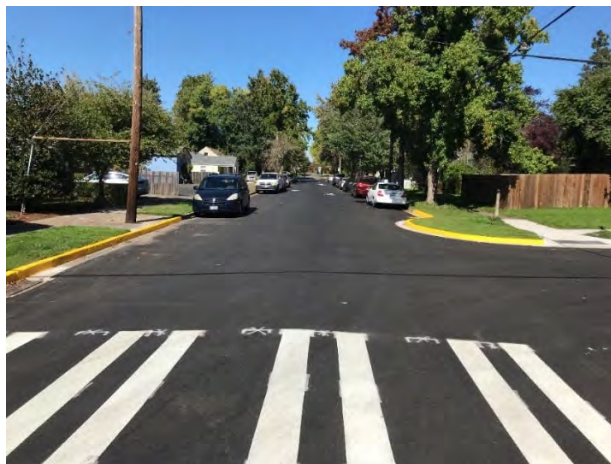
Completed Paving on Alder Street
