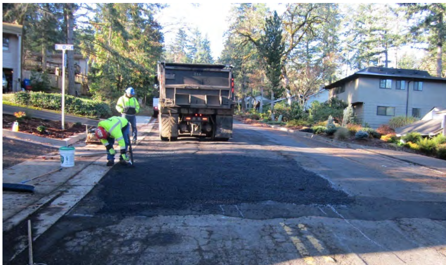
Brookside Street Temporary Paving for Winter
