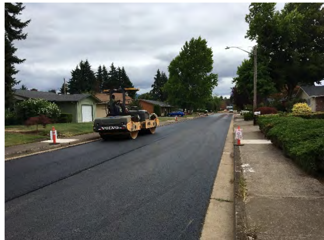
Paving on Balfour Street
