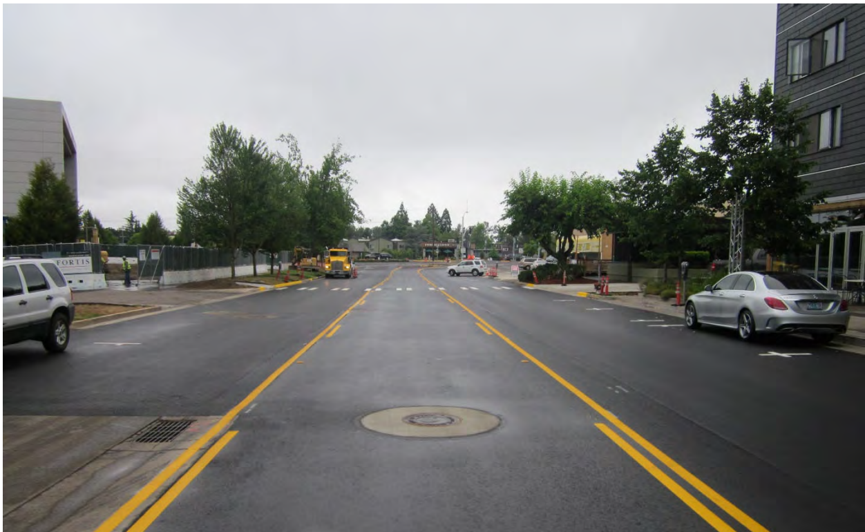
Completed Paving on Villard Street
