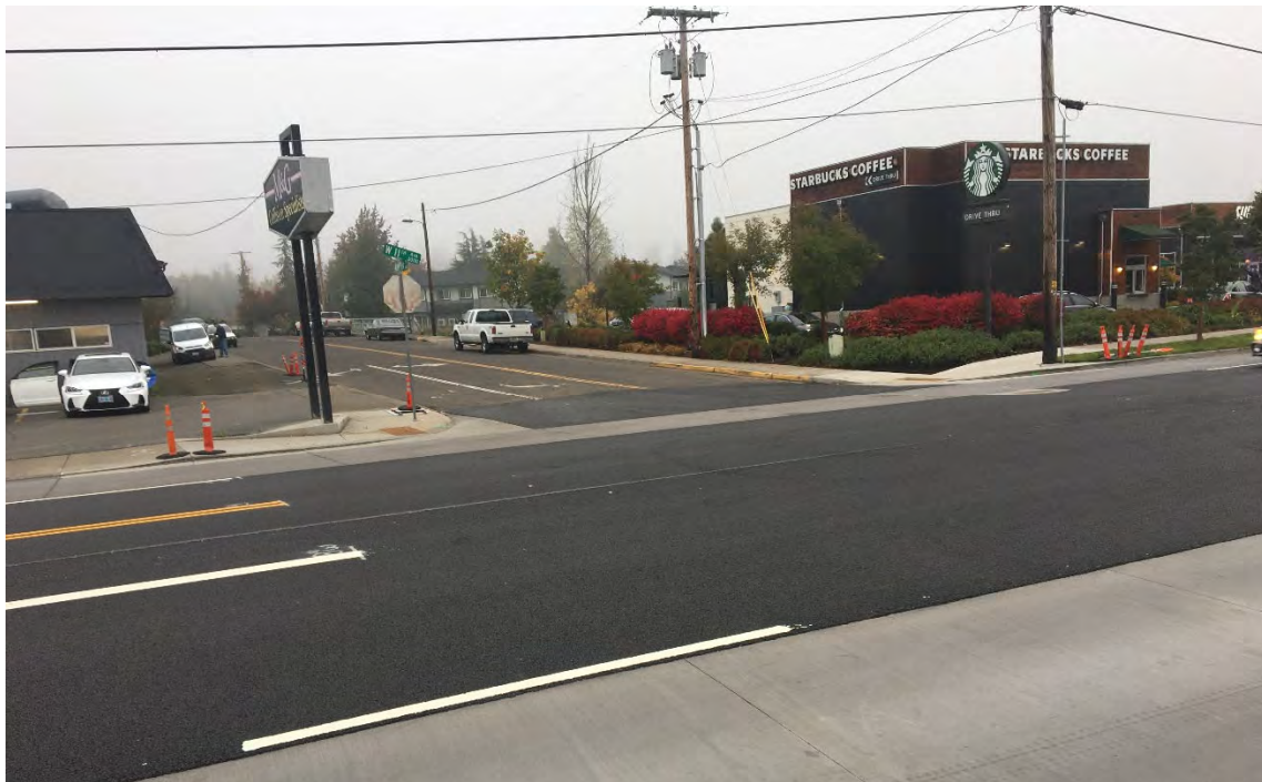
Completed Paving on W 11th Avenue
