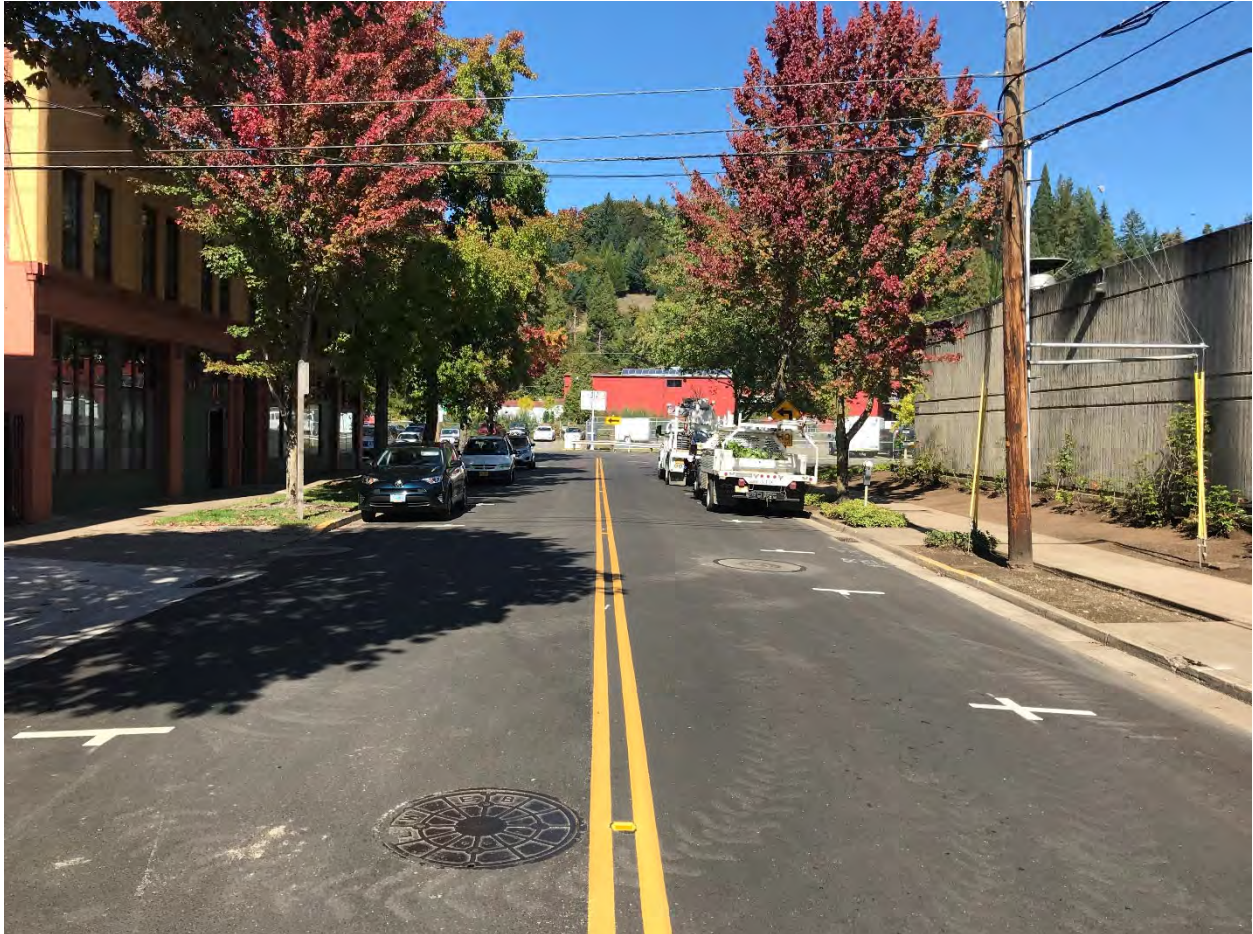
Completed 2019 Paving on Charnelton Street
