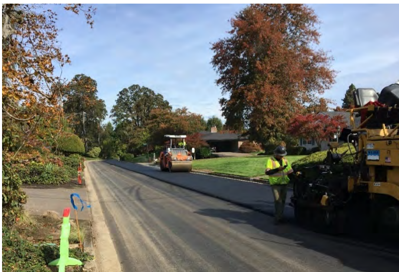
Paving on Fair Oaks Drive
