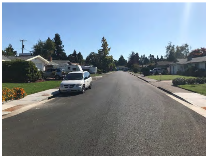
Completed Paving on Calgary Street
