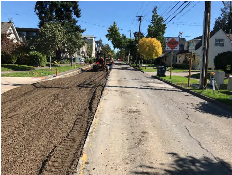
Ongoing Paving on East 19th Avenue
