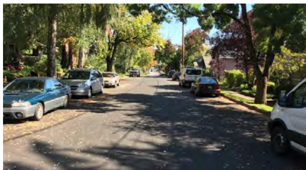
Completed Paving on 3rd Avenue
