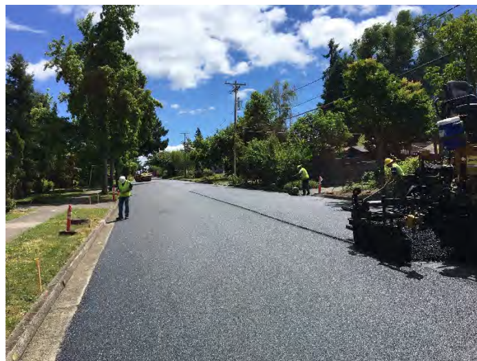
Paving on West 19th Avenue
