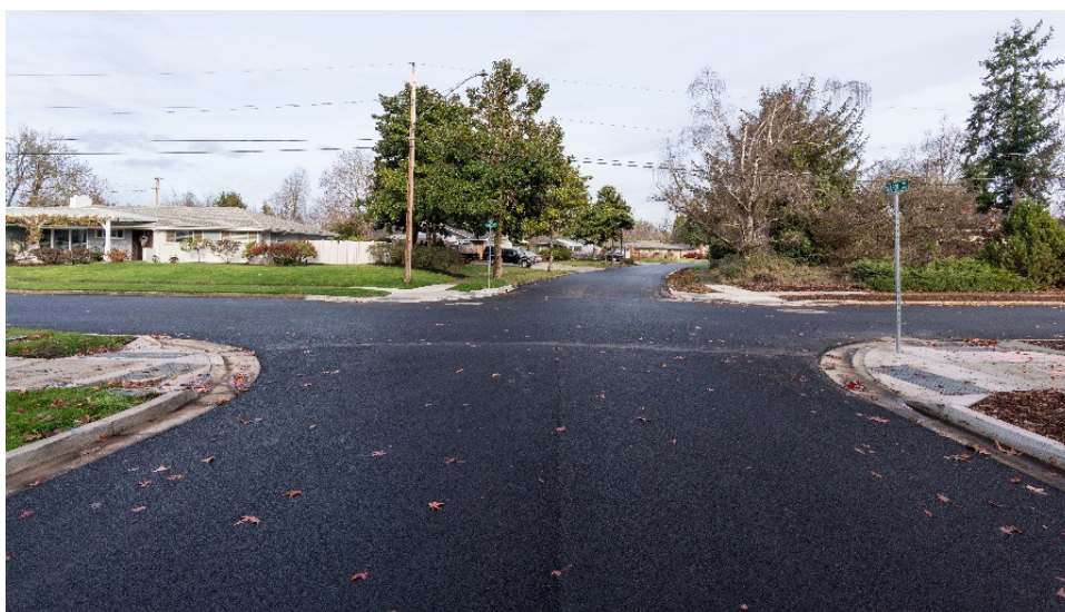
Completed Paving on Woodside Drive
