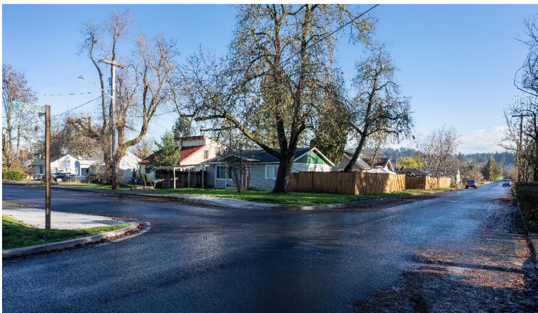
Completed 30th Ave Paving
