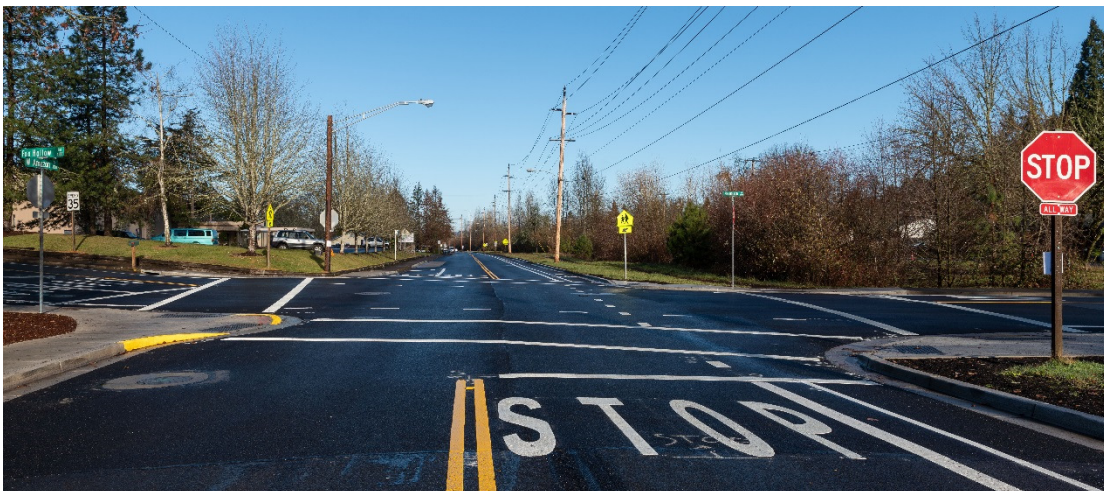
Completed Paving on W. Amazon Drive
