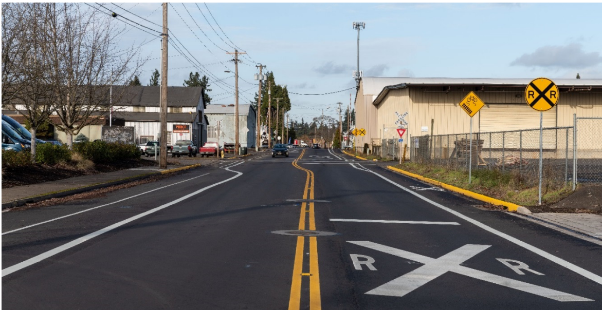
Completed Paving on Garfield Street
