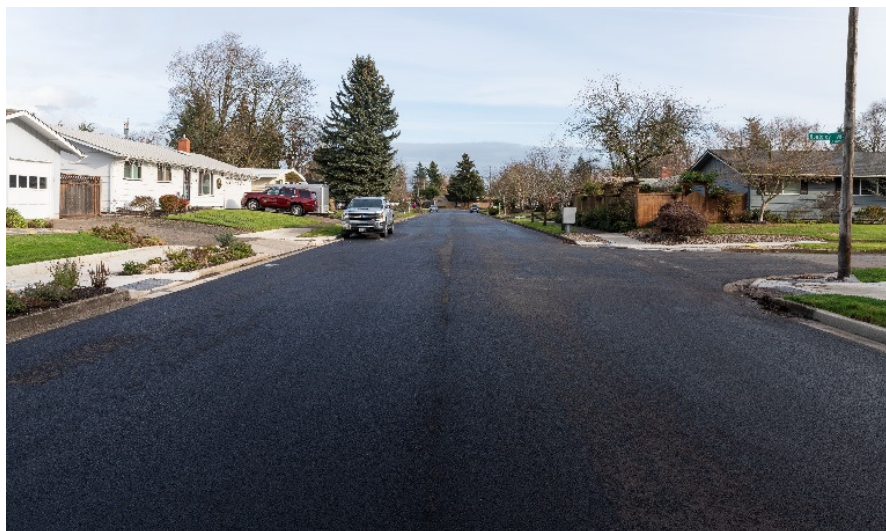
Completed Paving on Larkspur Ave
