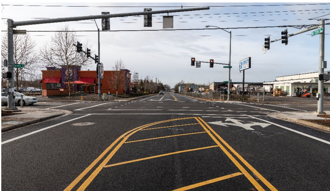
Completed Paving on 7th Place
