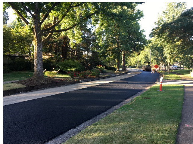
Paving on Woodside Drive
