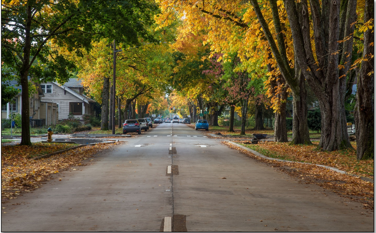
Completed 2017 Paving on Jefferson Street
