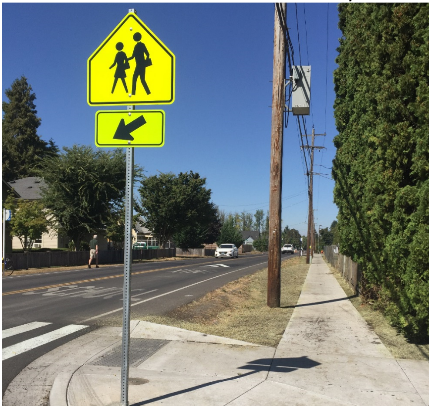
PIC #2: Sidewalk Infill and Crosswalk on N. Park Avenue by Howard Elementary
