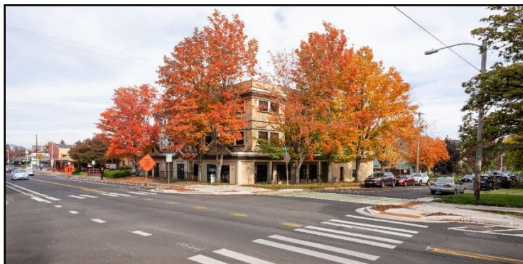
Completed Paving on 19 th Avenue
