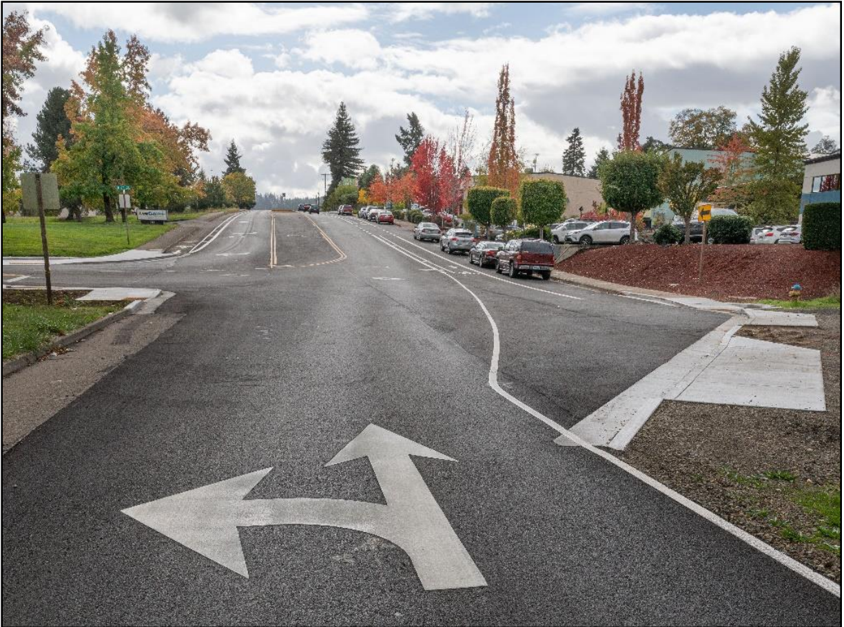
Completed Paving on Bailey Hill Road
