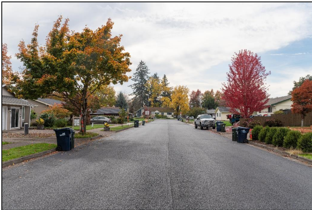
Completed Paving on Laurelhurst Drive
