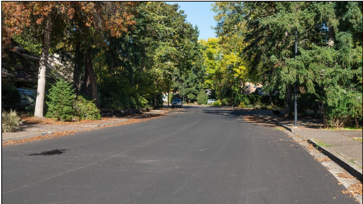
Completed Paving on Windsor Circle
