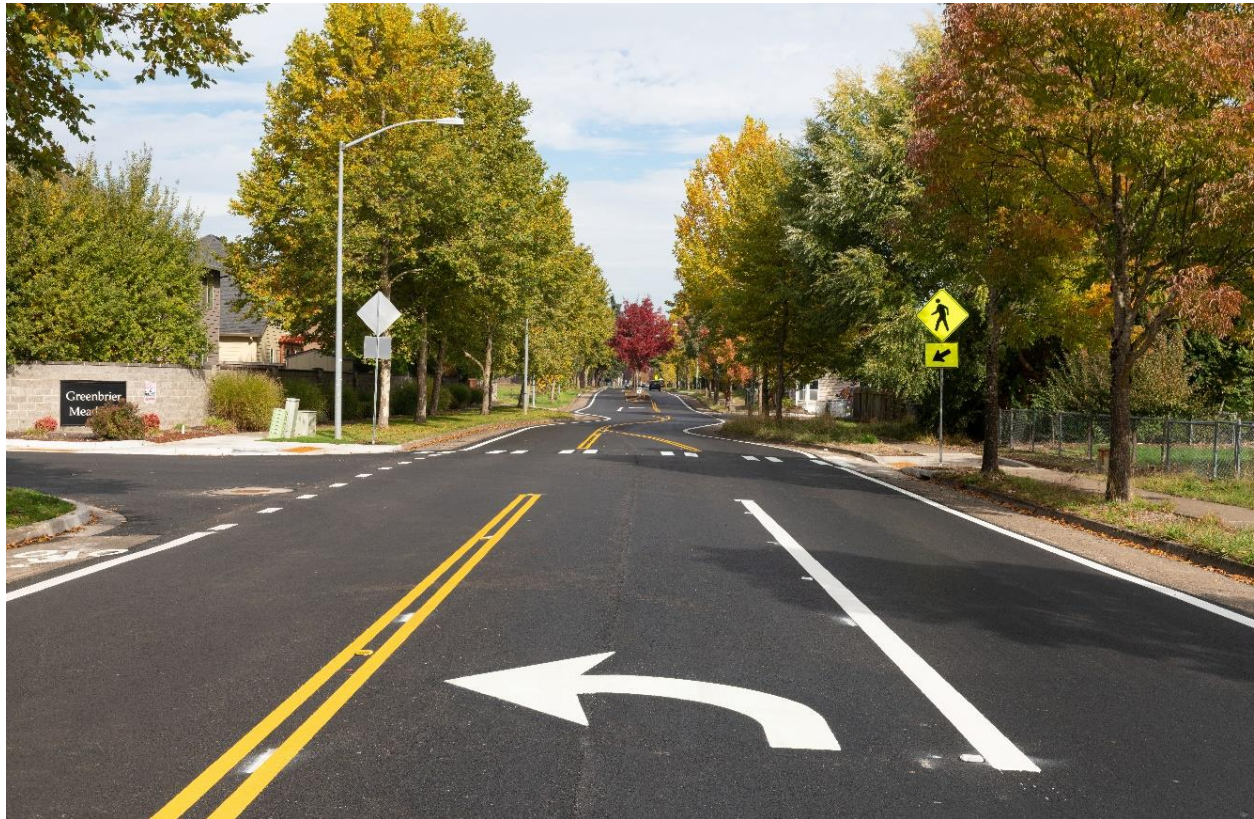
Completed Paving on Terry Street
