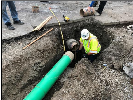
Stormwater Pipe Work on Primrose Street
