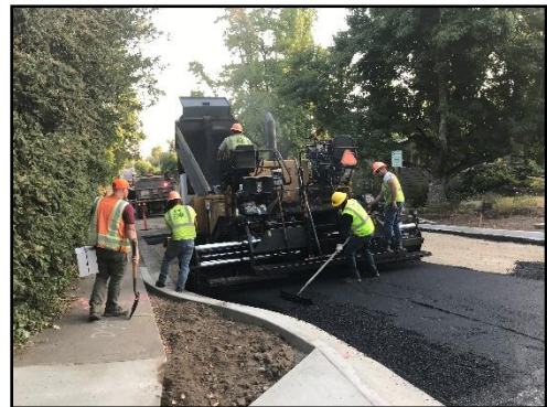
Paving on Fairmount Boulevard
