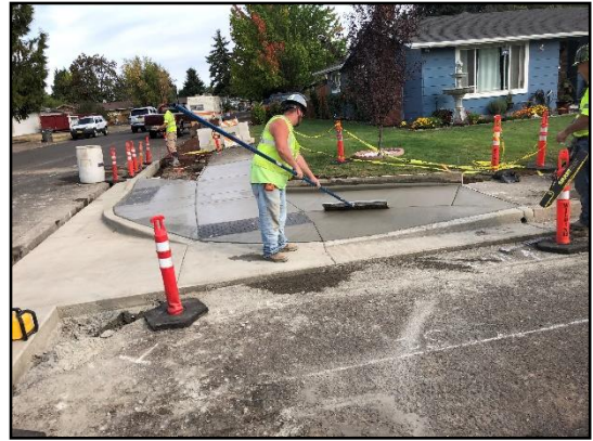
ADA Ramp Under Construction on Laurelhurst Drive
