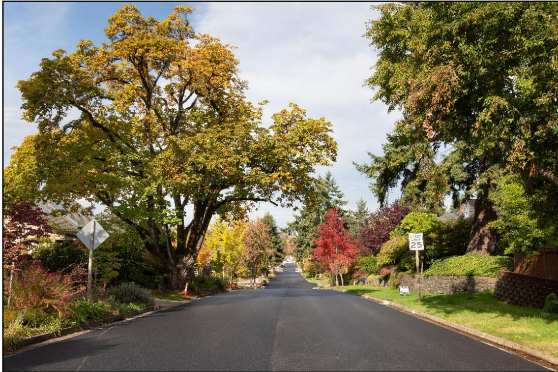
Completed Paving on Lincoln Street
