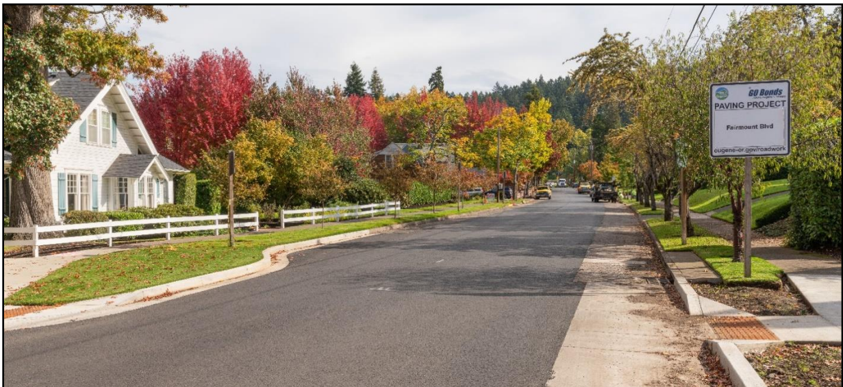
Completed Paving on Fairmount Boulevard
