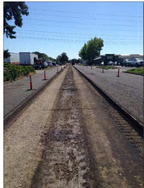
Pavement Removal on 5th Avenue
