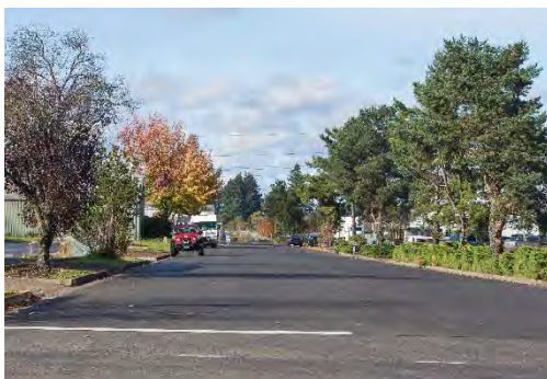
Completed Paving on 5 th Avenue
