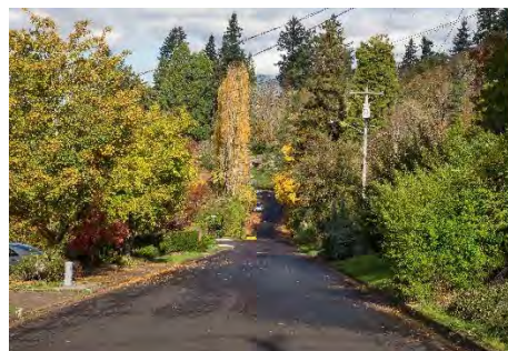
Completed Paving Van Ness Street
