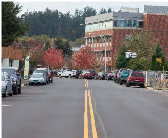
Completed Paving Centennial Loop
