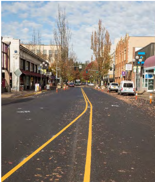
Completed Paving Willamette Street
