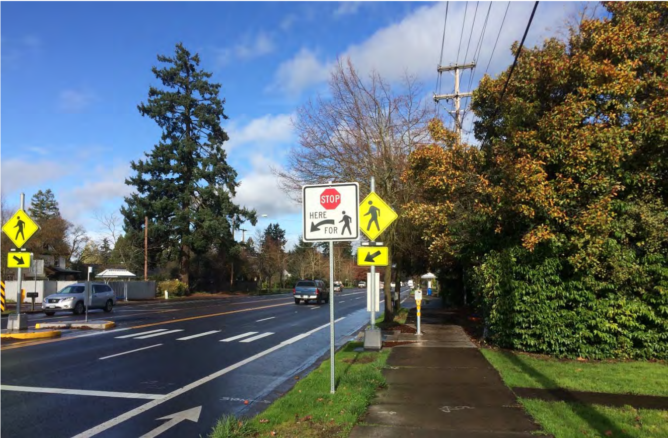
PIC #4: Fir Lane RRFB (River Road)
