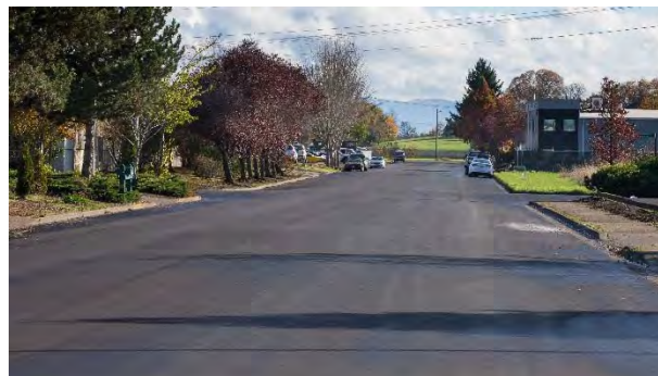
Completed Paving on 7 th Avenue
