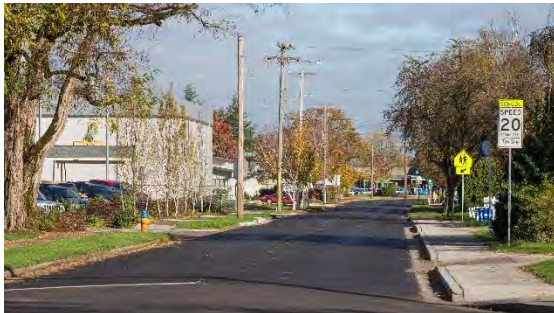
Completed Paving Fairfield Avenue
