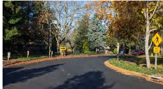
Completed Paving Jacobs Drive
