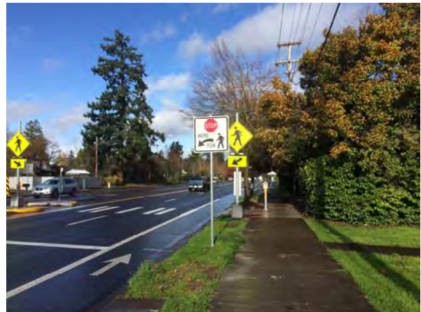
River Road RRFB
