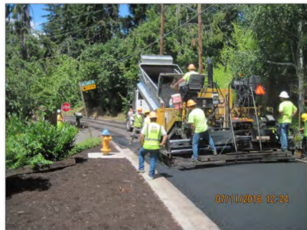
Paving on Spring Blvd
