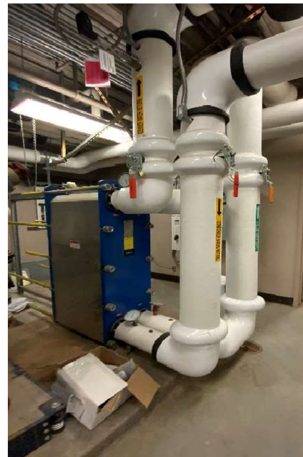
FIGURE 4-19 HEAT EXCHANGER DEDICATED TO WATER-SIDE ECONOMIZER
