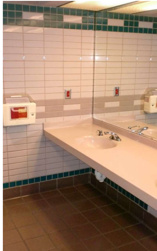
FIGURE 4-27 EXISTING LAVATORY AT LANESIDE RESTROOM
