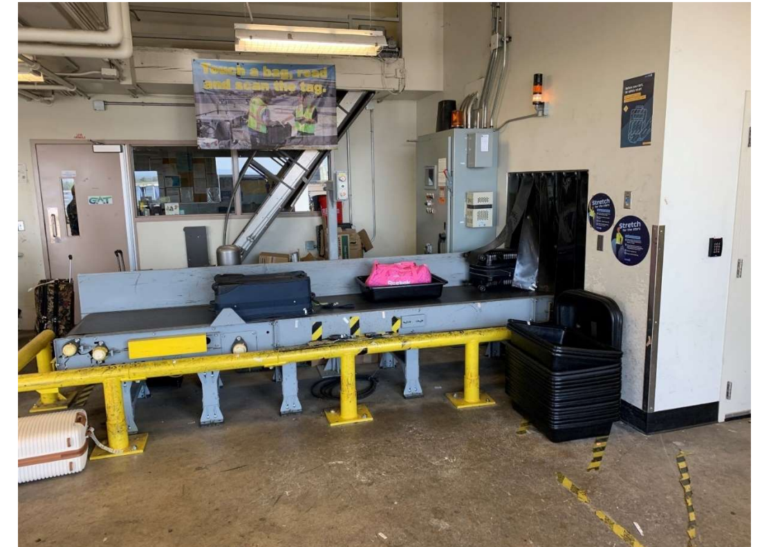
FIGURE 4-41 TC4 MAKE-UP AREA
