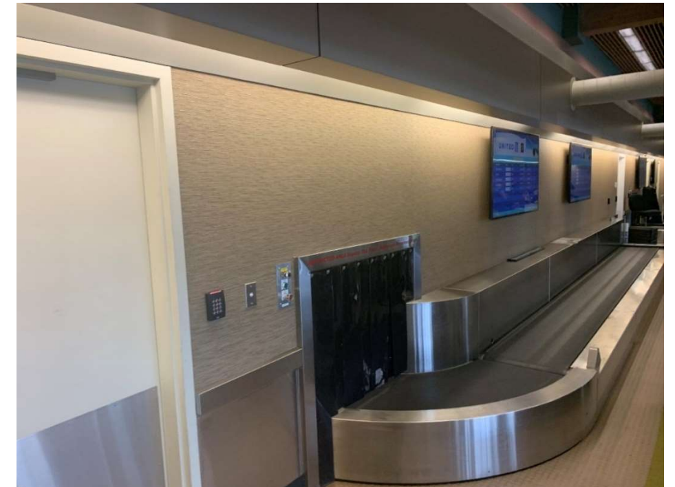
FIGURE 4-31 TICKETING LOAD BELT TC4
