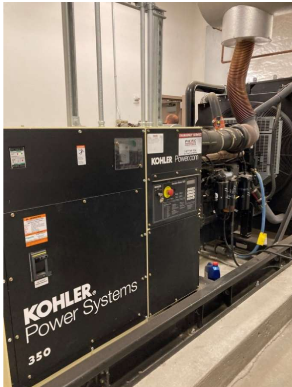
FIGURE 4-24 EMERGENCY GENERATOR
