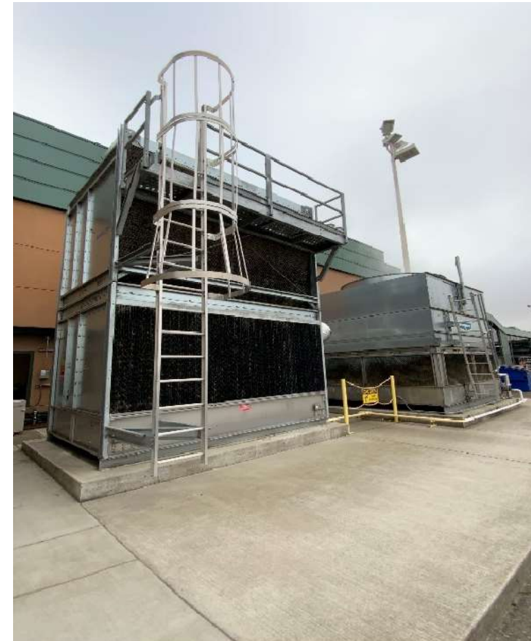
FIGURE 4-20 FLUID COOLERS AT CONCOURSE A
