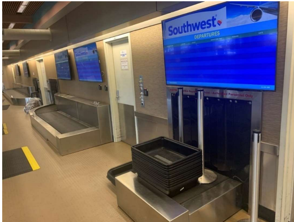
FIGURE 4-29 TICKETING LOAD BELTS TC1, TC2, AND TC3
