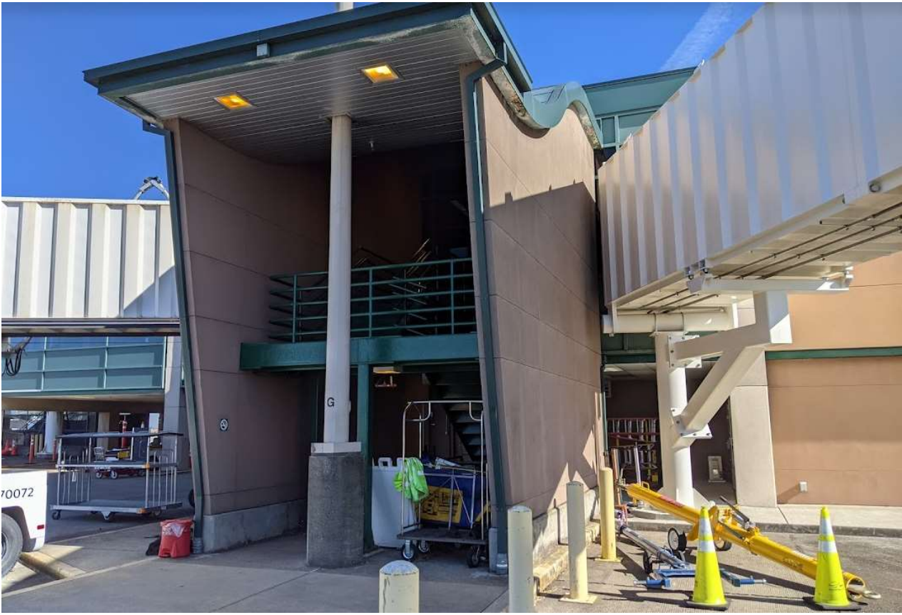
FIGURE 4-9 OPEN STAIR ENTRANCE
