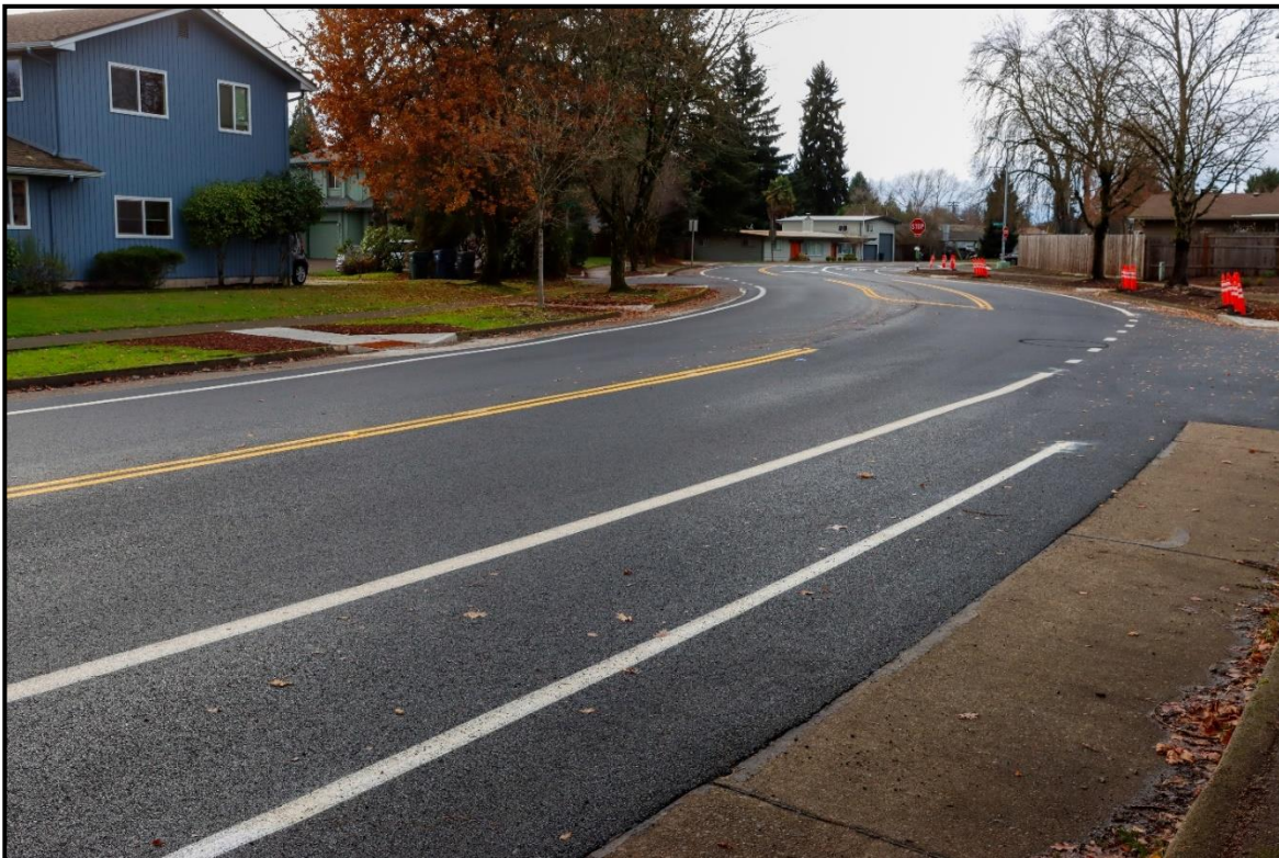
Completed Paving on Crescent Avenue
