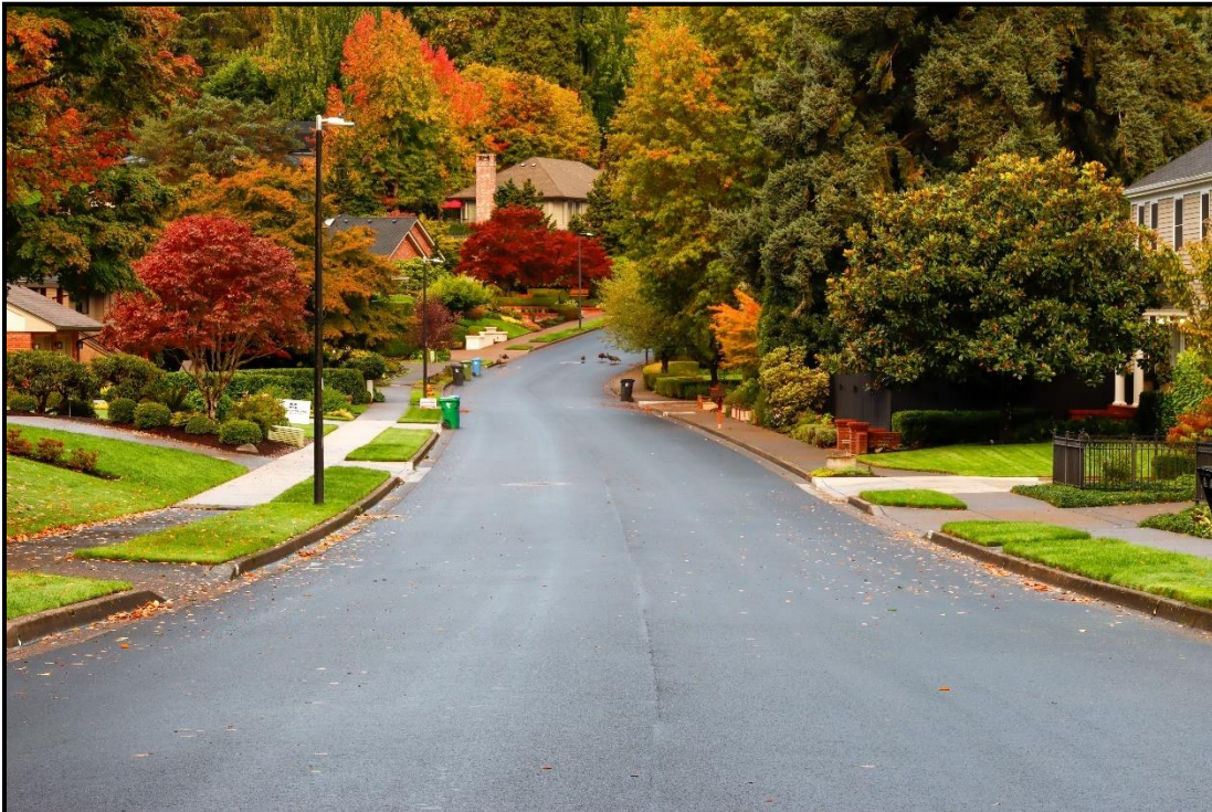
Completed Paving on Spyglass Drive
