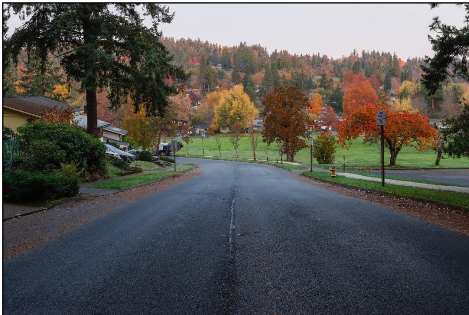
Completed Paving on 46 th Avenue
