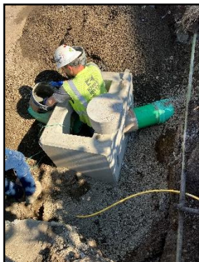
Stormwater Pipe Work on Polk St
