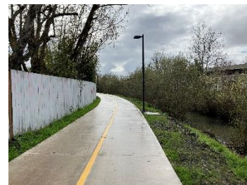
Completed repairs to the Fern Ridge Path
