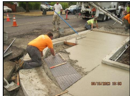
ADA Ramp Under Construction on Chambers Street
