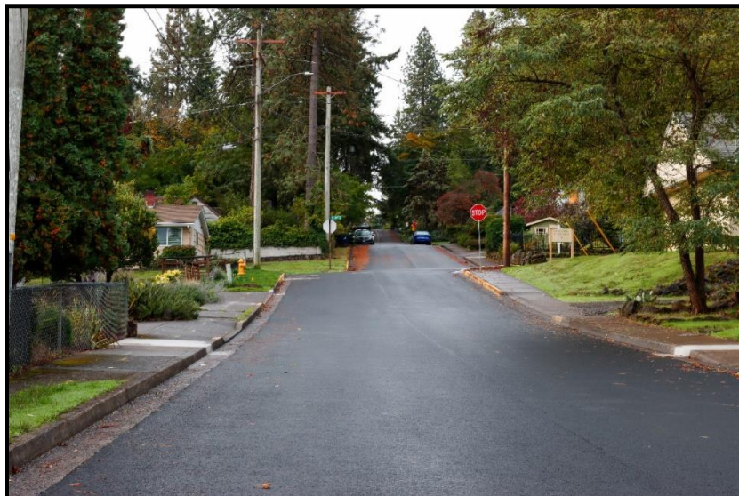
Completed Paving on Portland St
