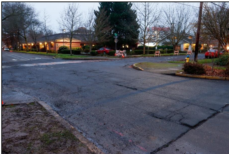
Existing Pavement Condition on Oak Street
