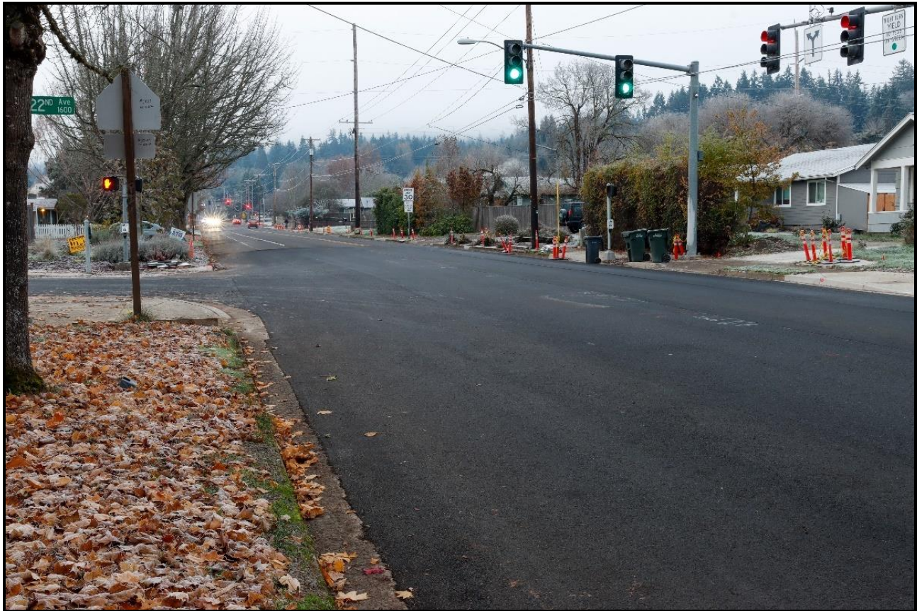
Completed Paving on a Chambers St Intersection
