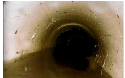
Lined concrete pipe with sealed joints.
