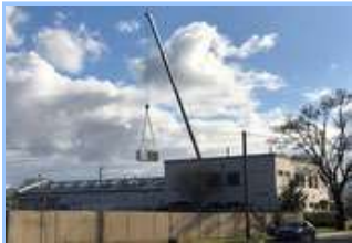
Installing a new HVAC unit for the building.
