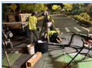
Lining a wastewater pipe
