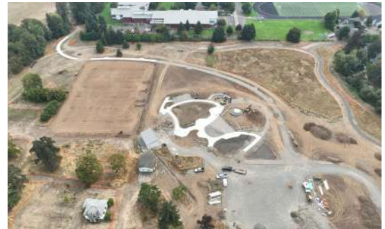
Santa Clara Community Park under construction
