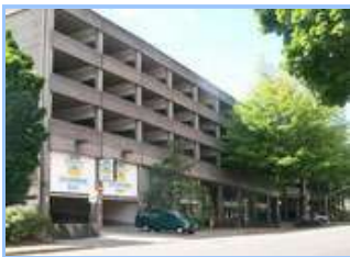
Downtown Eugene, Overpark Parking Garage - 1000 Oak St.
