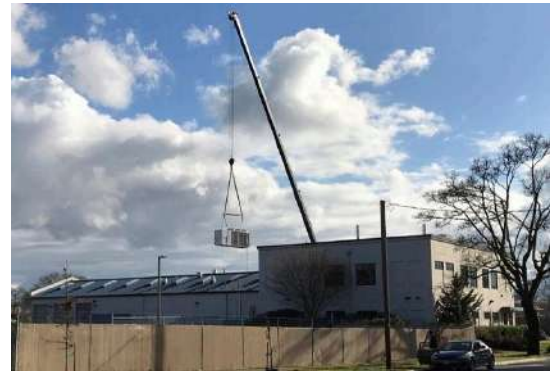
Eugene Police Services Building
