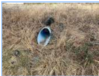
Tip up stormwater pipe
