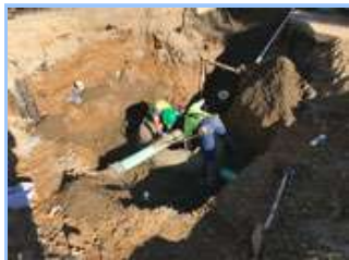
Wastewater pipe replacement
