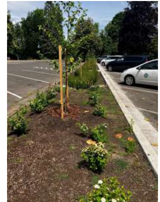
Vegetated rain gardens at Skinner Butte Park
