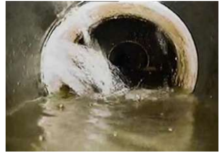
Concrete pipe with excessive groundwater flowing in through open pipe joints.
