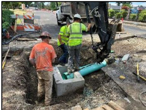
Stormwater Pipe Work on Bailey Lane
