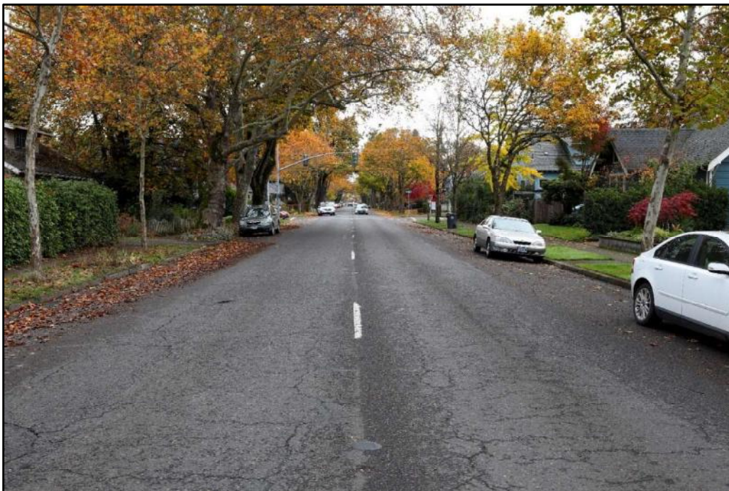
Existing Pavement on W 11th Avenue
