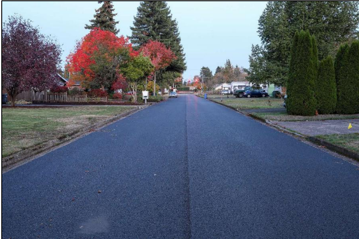
COMPLETED PAVING ON CARMEL AVENUE
