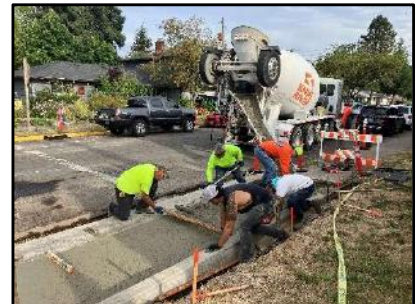
ADA Ramp Under Construction on Carmel Avenue
