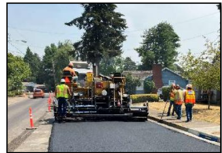
Paving on Bailey Lane
