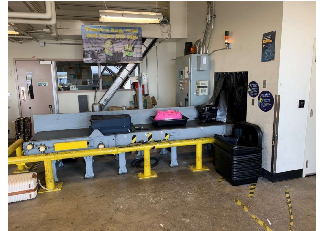
FIGURE 4-40 TC4 MAKE-UP AREA
