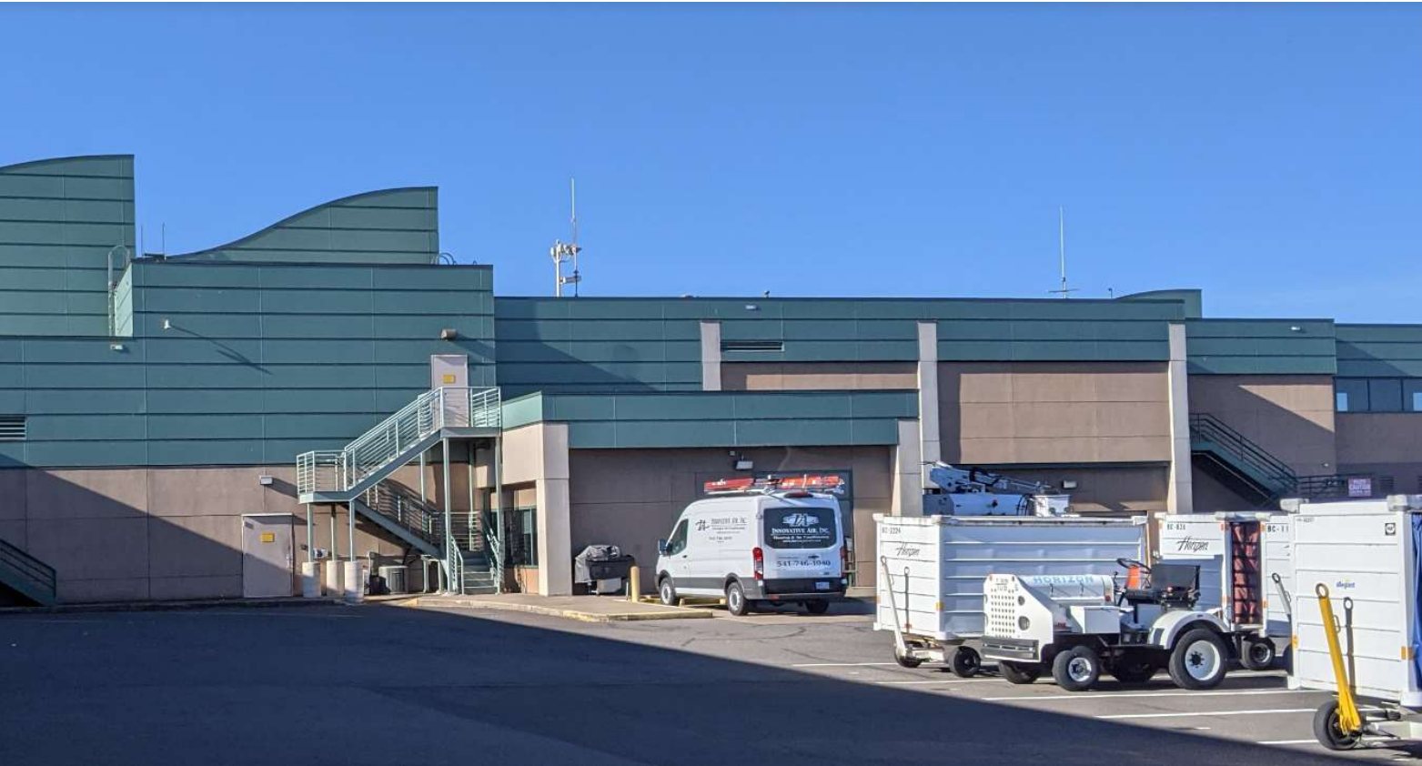
FIGURE 4-8 TYPICAL AIRSIDE EXTERIOR FINISHES
