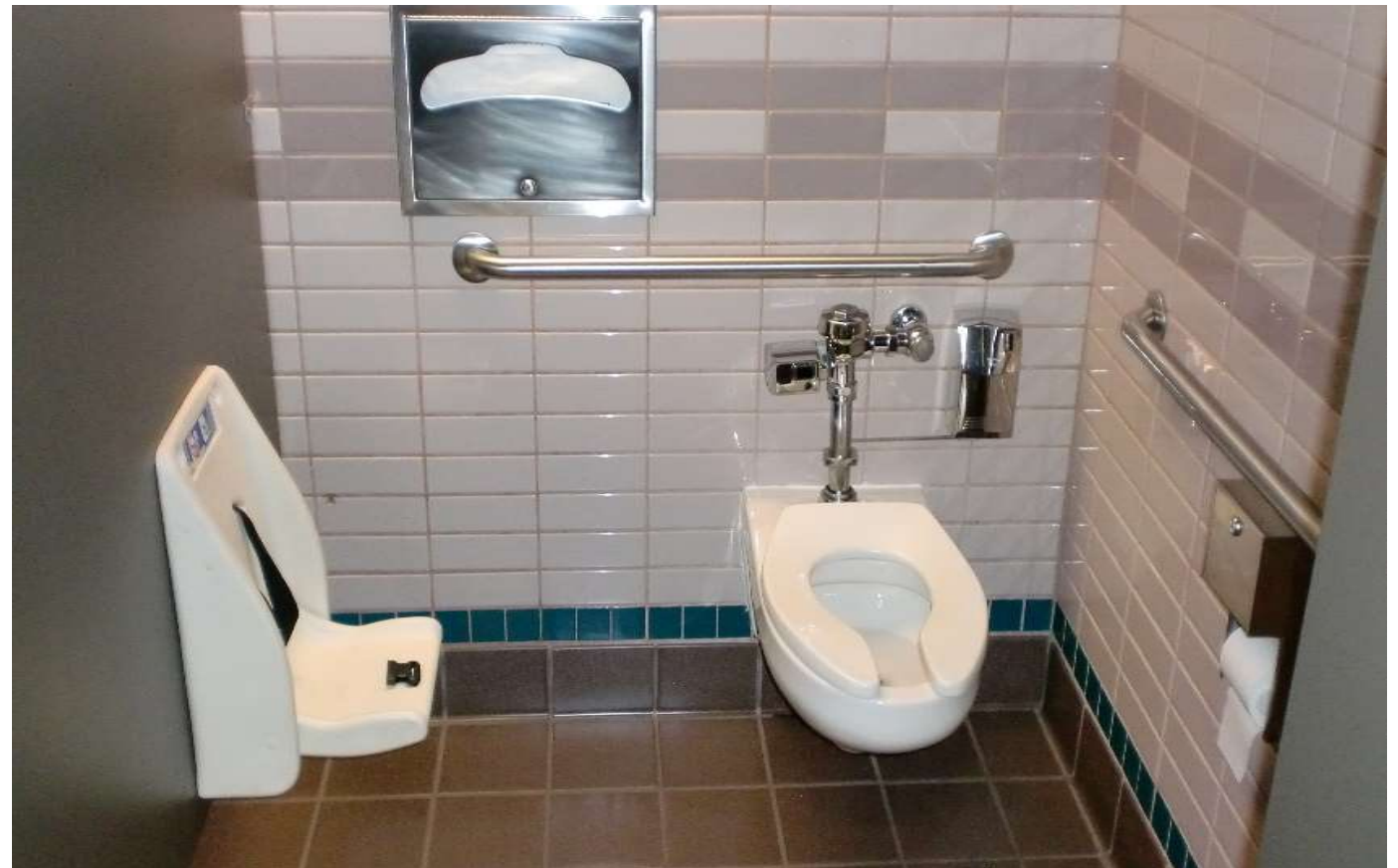
FIGURE 4-28 EXISTING WC AT LANDSIDE RESTROOM
