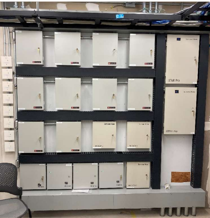
FIGURE 12-10 EXISTING WALL-MOUNTED SECURITY EQUIPMENT IN MDF
