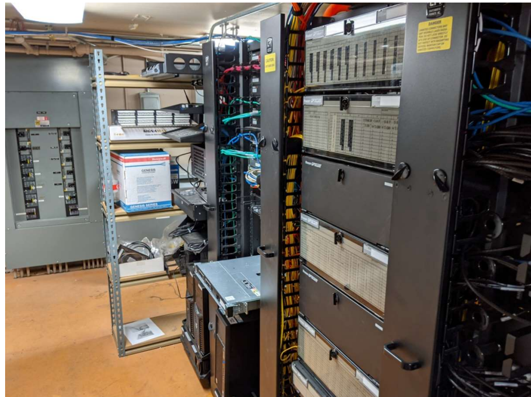
FIGURE 4-25 COMM ROOM ABOVE BAGGAGE HANDLING
