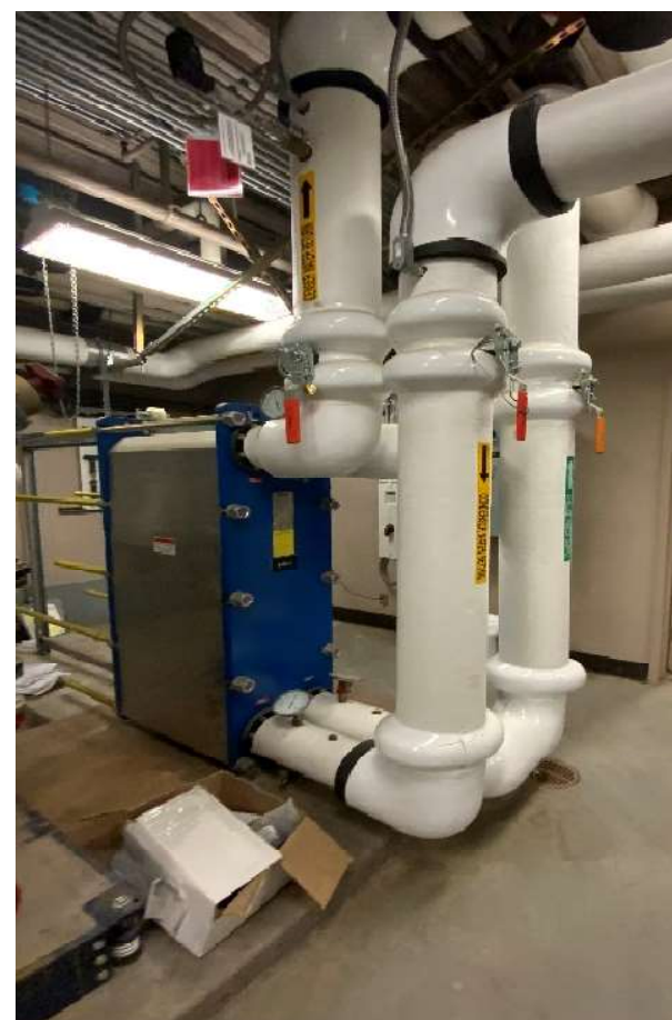
FIGURE 4-19 HEAT EXCHANGER DEDICATED TO WATER-SIDE ECONOMIZER
