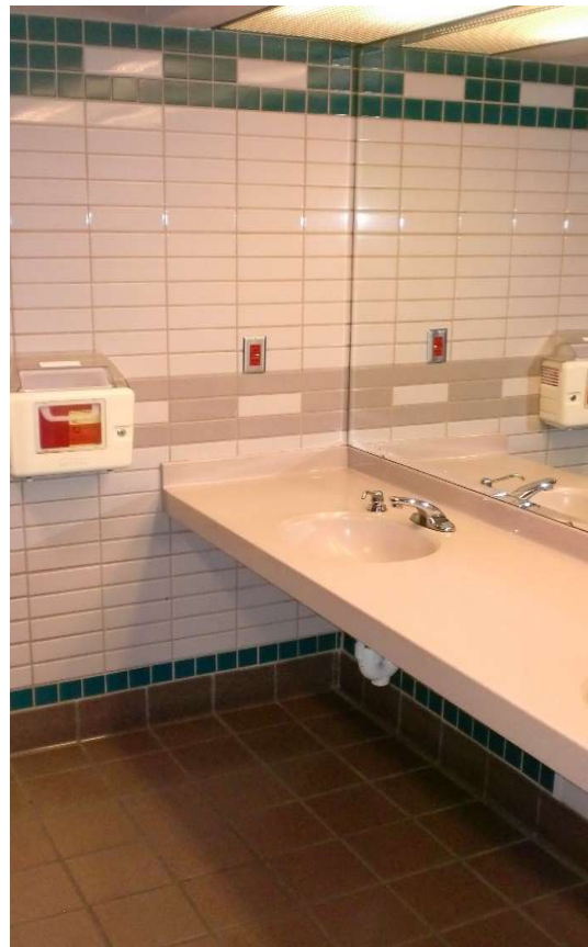
FIGURE 4-27 EXISTING LAVATORY AT LANDSIDE RESTROOM
