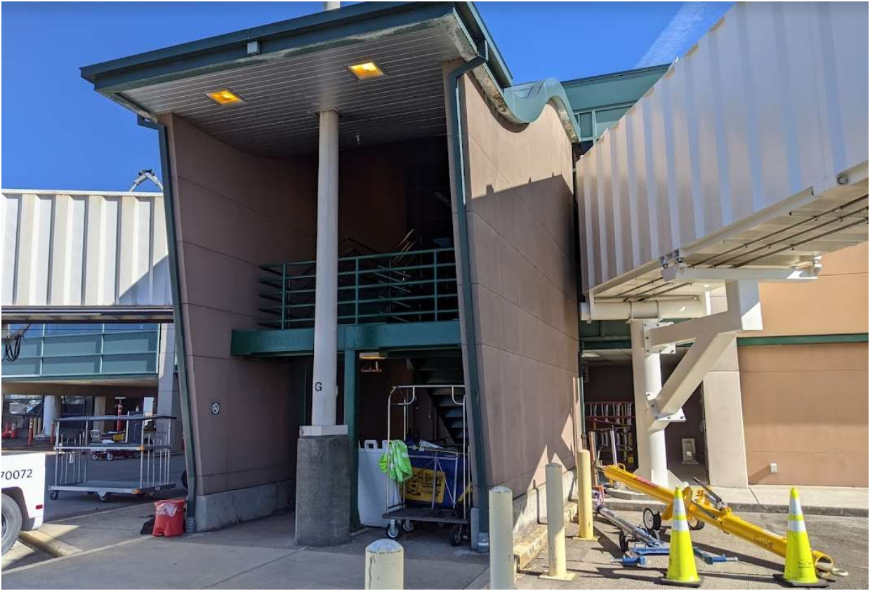
FIGURE 4-9 OPEN STAIR ENTRANCE
