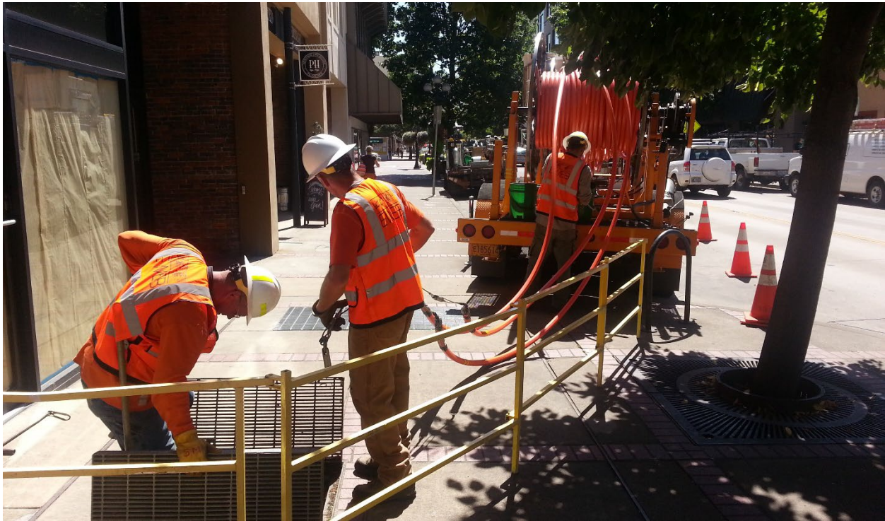
Microduct installation in Downtown Eugene. Photo by City of Eugene staff.
