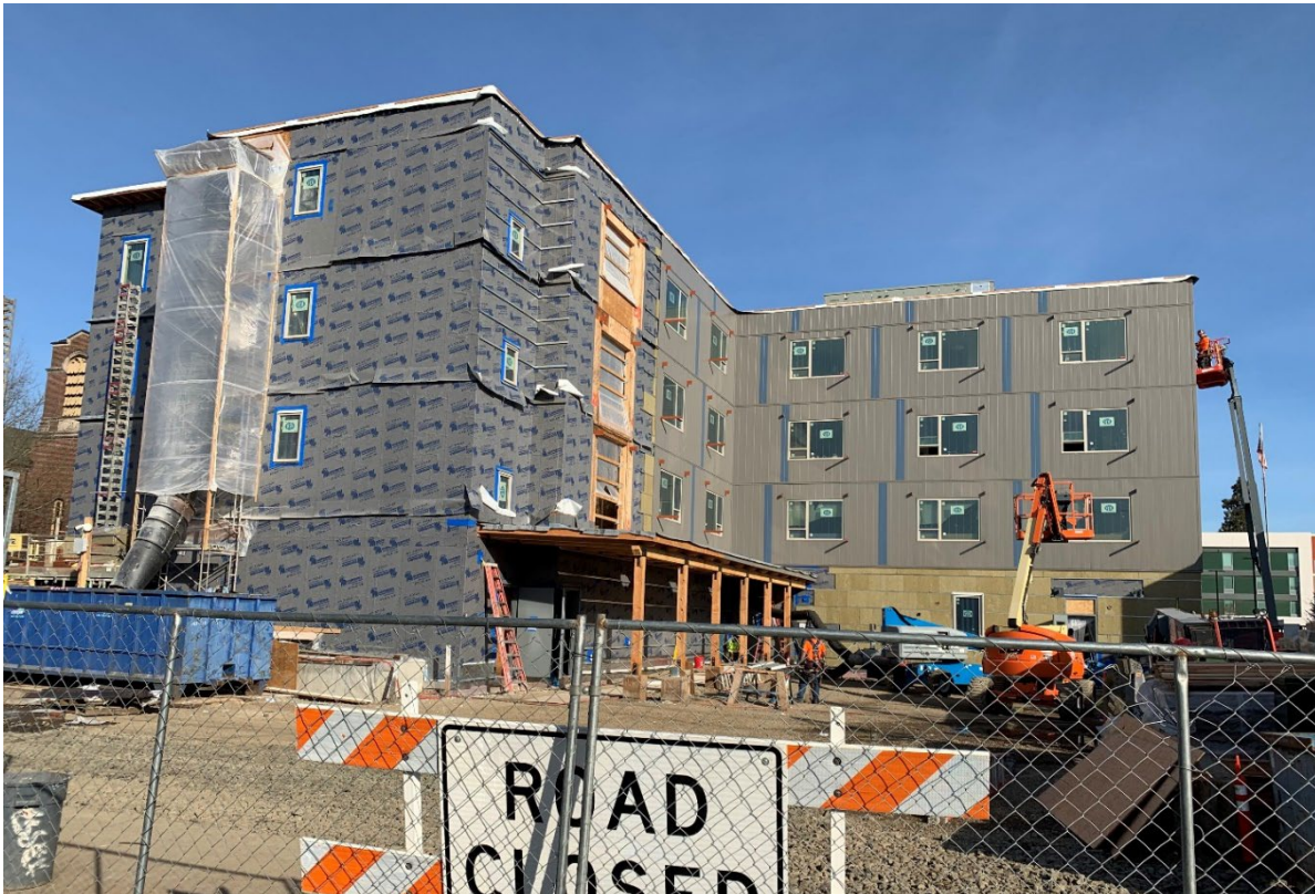
Development of The Nel (Permanent Supportive Housing). Photo by City of Eugene staff.
