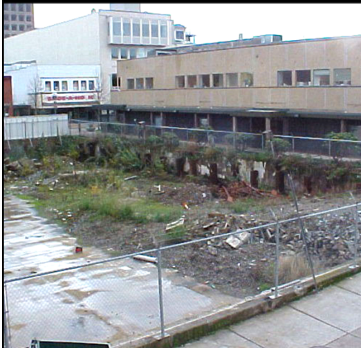
Supported new Woolworth Building on Willamette Street, filling an empty pit
