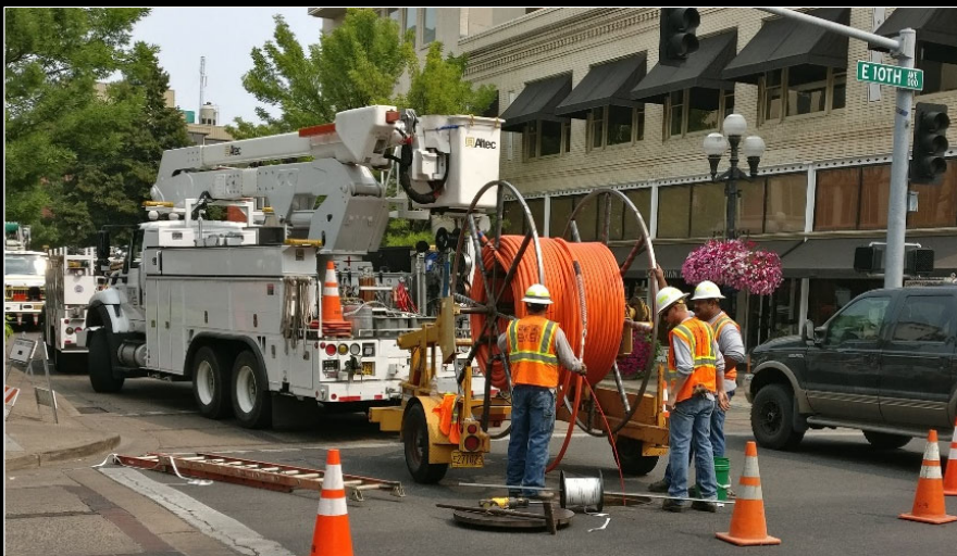
Installation of microduct for fiber project
