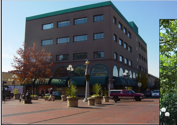
Center Court building renovated into the Broadway Commerce Center
