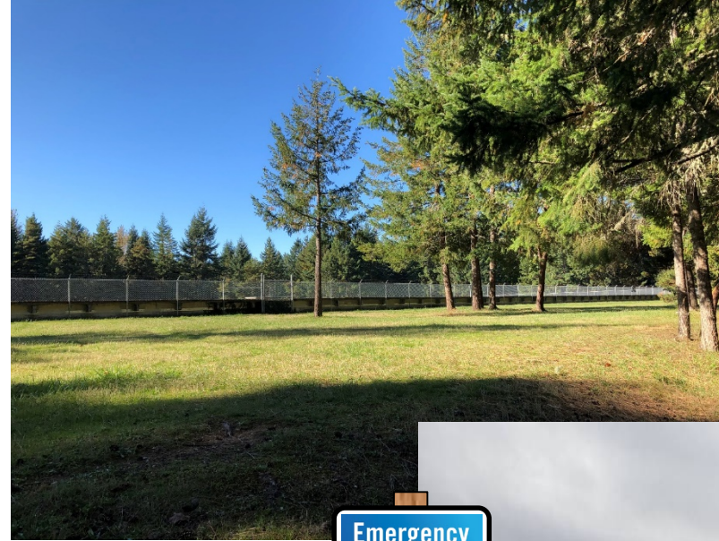
Hawkins Hill Reservoir
