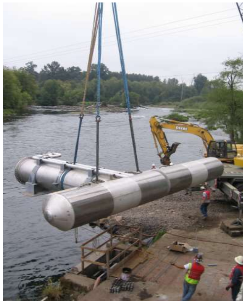
New Hayden Bridge Intake
