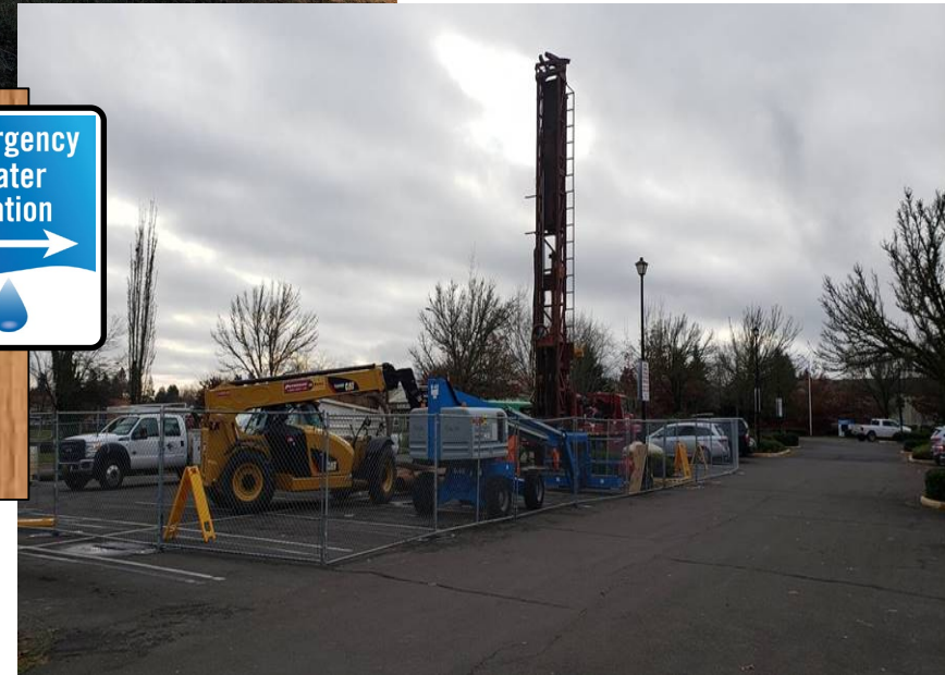
Emergency Well Drilling – Sheldon Fire Station
