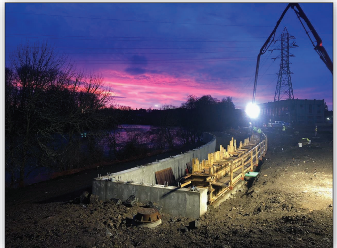
Downtown Riverfront Park Construction Monday 1/11/2021, 6:30 a.m.
