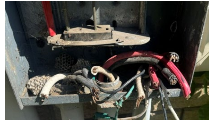
Upper images: Electric service disconnected at the pole; master meter removed. Lower images: Electric service cut at the breaker box; breaker panel in poor condition
